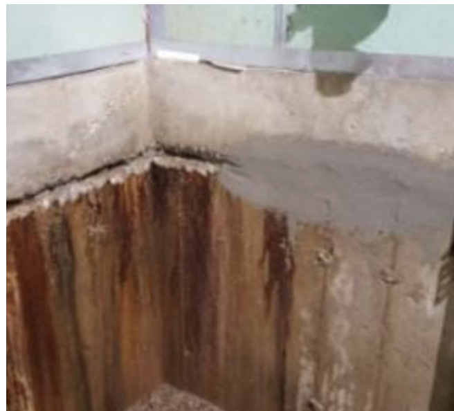
The active leaks, cracks and joints treated with Xypex Patch'n Plug.
