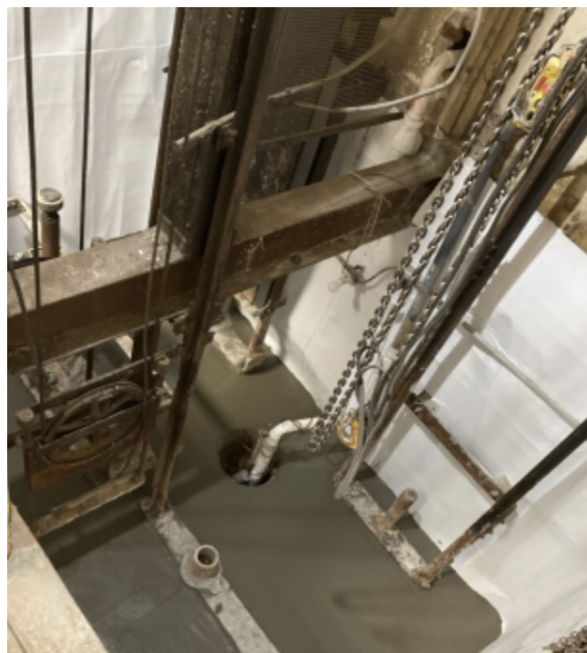
A half-inch layer of Megamix II was also applied to create a durable, smooth, strong and waterproof floor.
