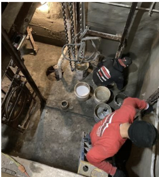
Two coats of Xypex Concentrate slurry were then applied to the floor and walls.
