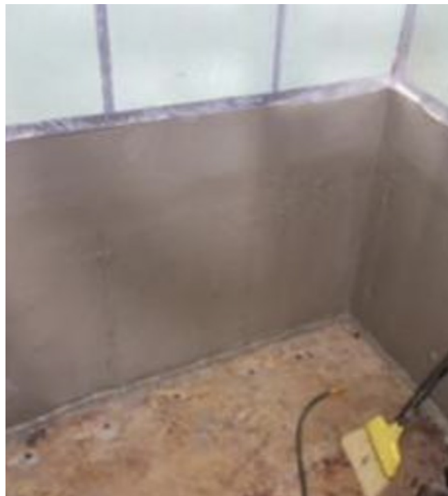
A layer of Xypex Megamix I was applied to the walls for added protection.
